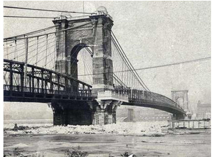
courtesy of www.roeblingbridge.org
