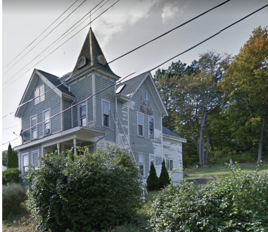
A Google Maps view of 72 (now 83) Powow Street undergoing renovation.
